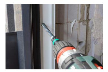
Determine the length of screw required:
